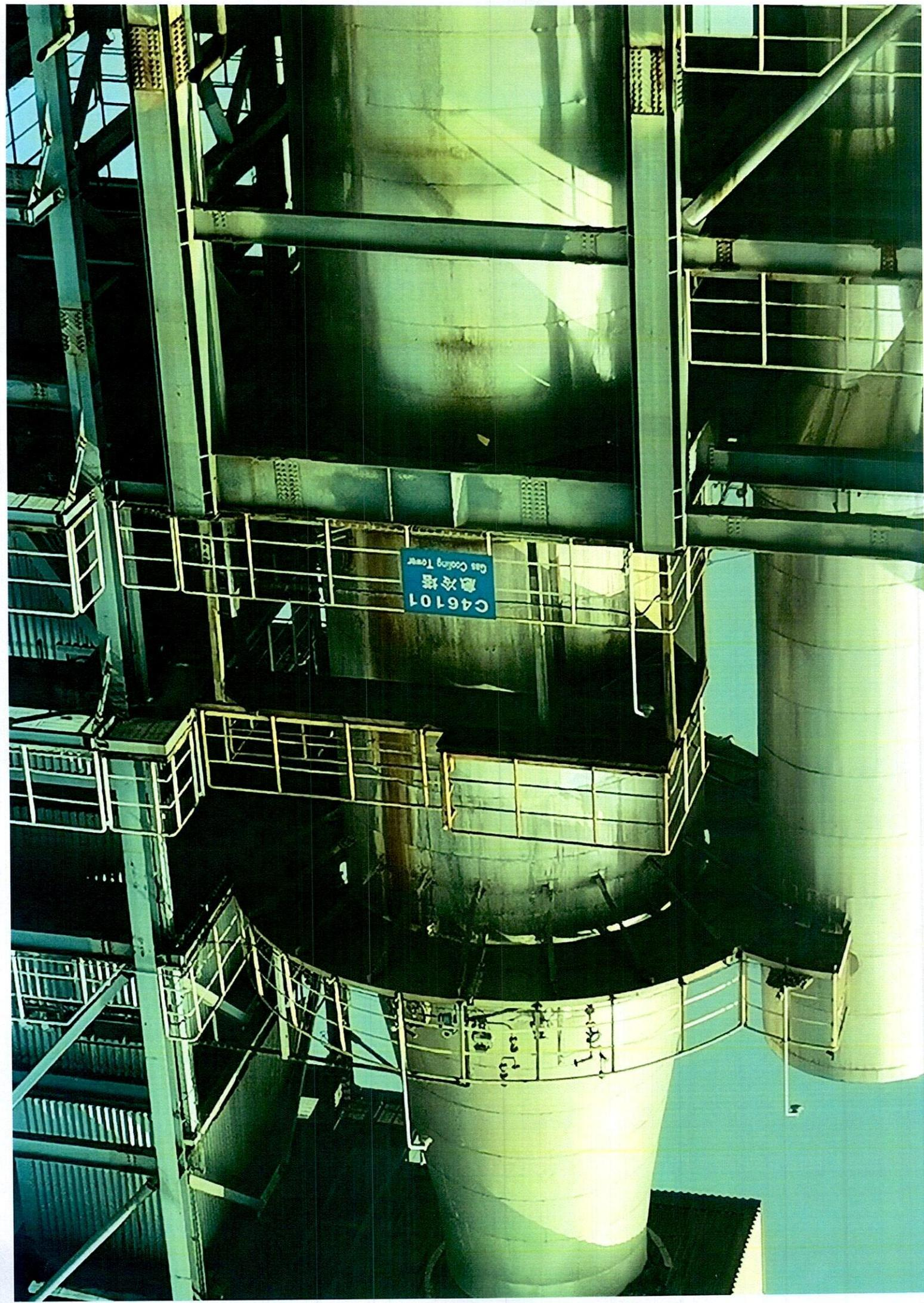
C46101 氣冷塔 Gas Cooling Tower
